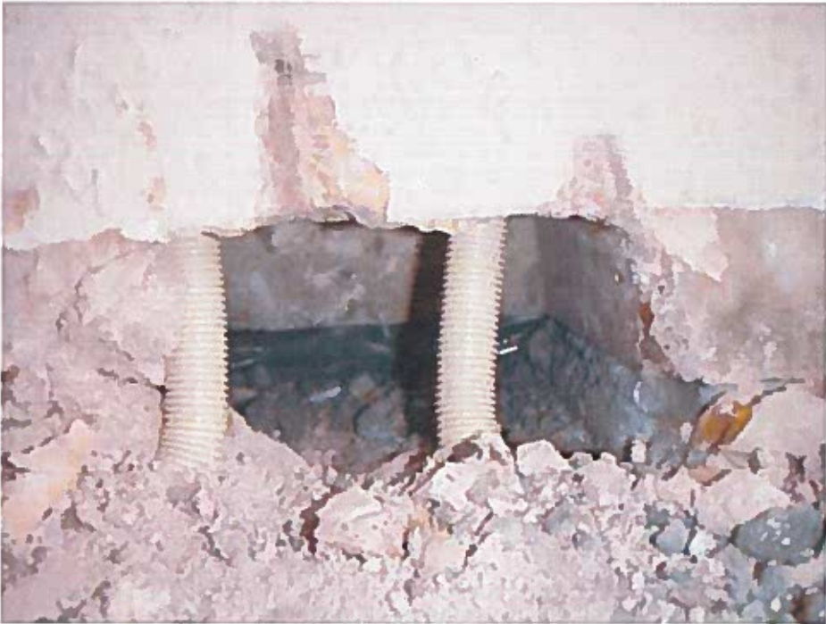
Photograph 13 Breakout L8 Air-filled compressible fill material at rear of panel
