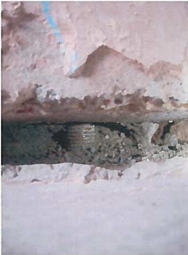
Photograph 16 Breakout L9 Shim observed in void beneath panel
