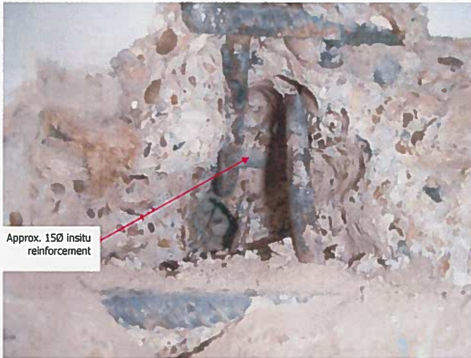
Photograph 19 Breakout U2 tying reinforcement at wall – soffit joint at first floor
