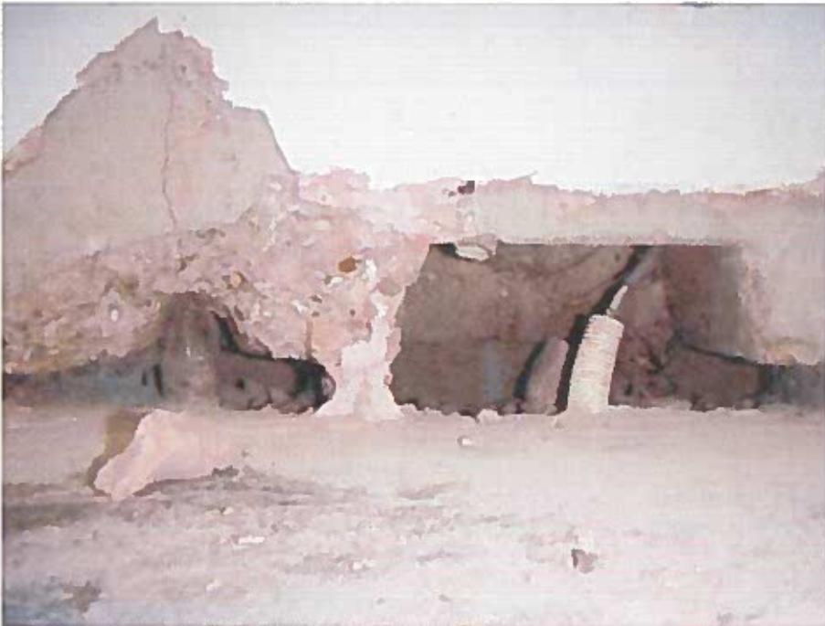
Photograph 2 Breakout L1 Dowel bar and service void rebate (typical)
